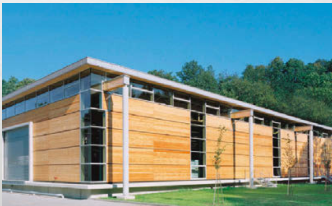
NiroSan® Press stainless steel fitting plant in Schmedefeld near Dresden
