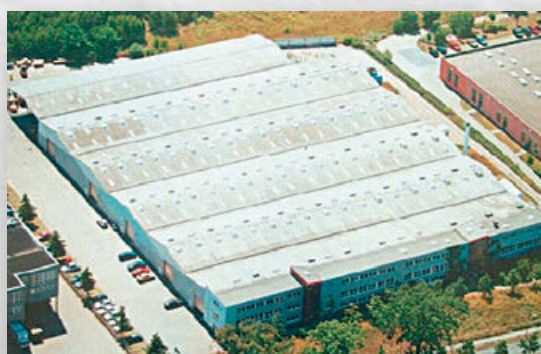
NiroSan® stainless steel pipe plant in Berlin
